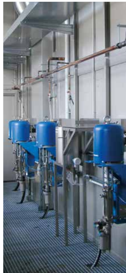
Plant construction and installation
